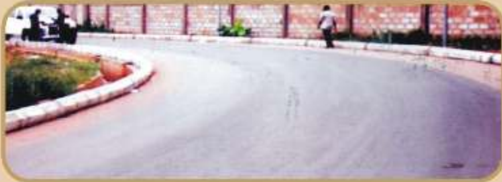
REHABILITATED OMORUYI STREET
