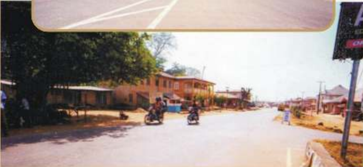
RECONSTRUCTED IGARA ROAD
